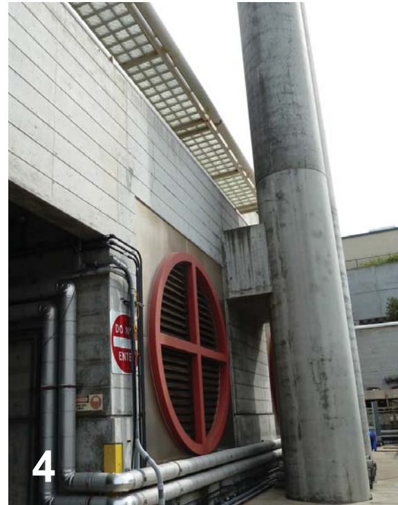
EXISTING MECHANICAL BLDG. SUPPLY & EXHAUST
