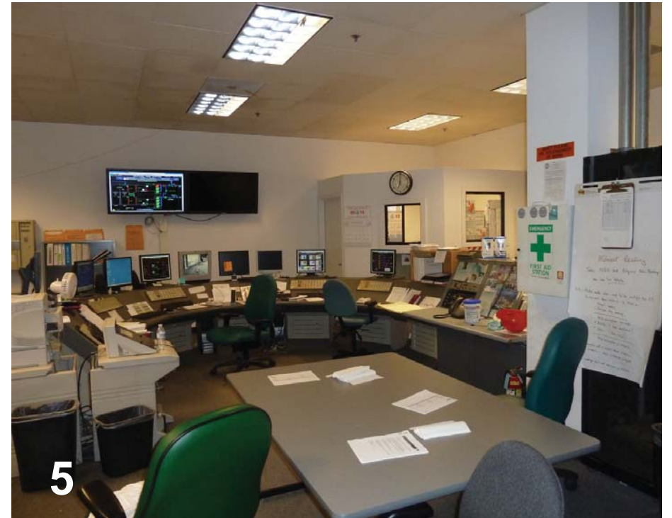
EXISTING UNDERGROUND CONTROL ROOM
