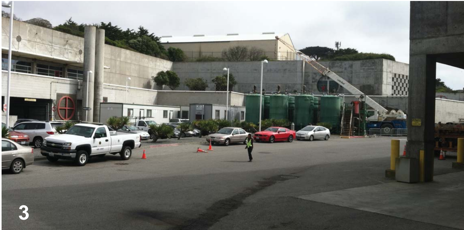
EXISTING TRAILERS AND BIOFUEL TANKS
