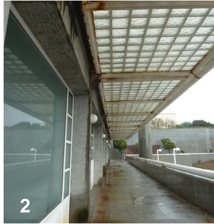
PEDESTRIAN WALKWAY AT ADMIN. BUILDING
