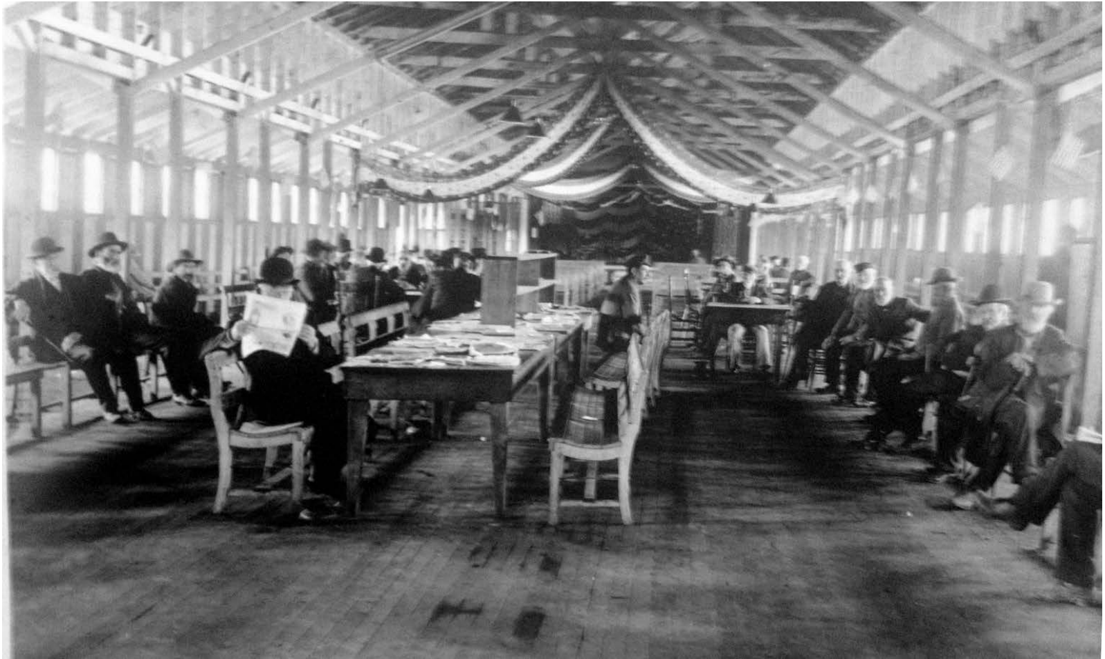
'08 Earthquake Shelter in Ingleside Track Horse Barn
