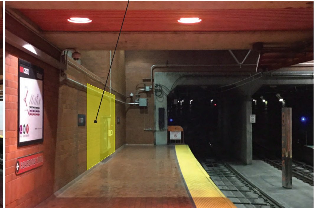
New opening for elevator exit
