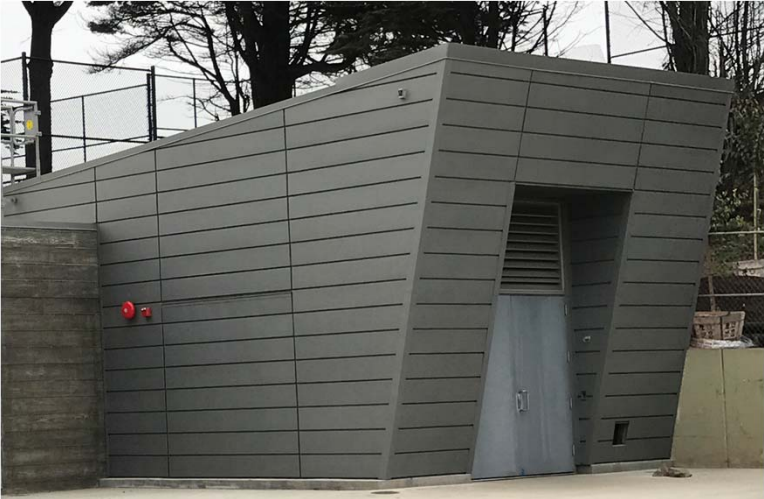
SFPUC WEST SUNSET PUMP STATION
