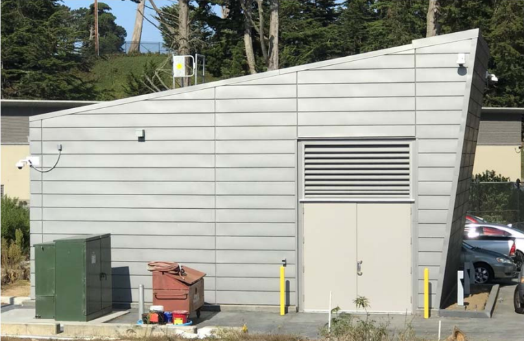
SFPUC LAKE MERCED PUMP STATION
