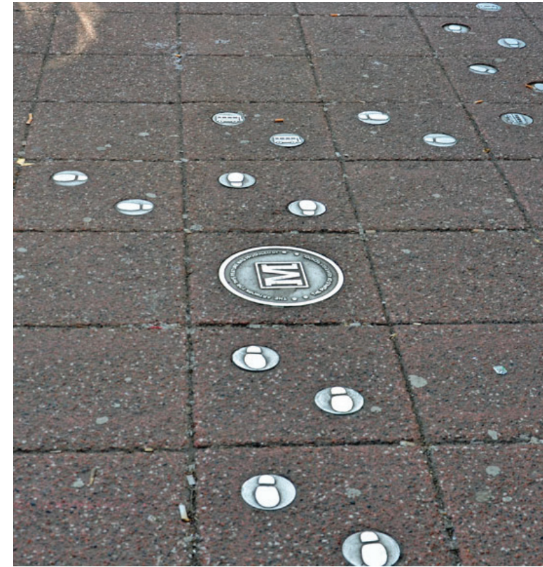
Flush stainless steel studs and dedication plaques in paving
