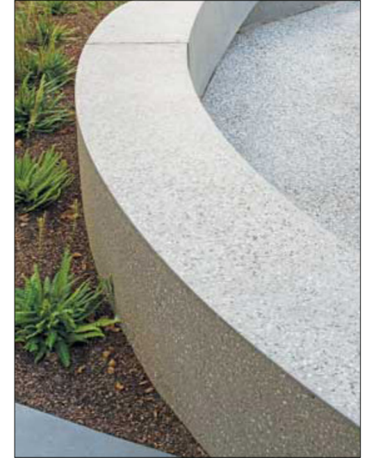
cast-in-place concrete seatwall planters
