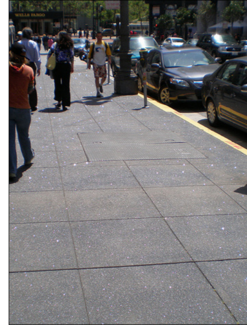
Silicon carbide grit finish paving
