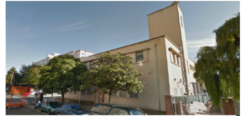
TURK STREET - NORTH & WEST FACADES
