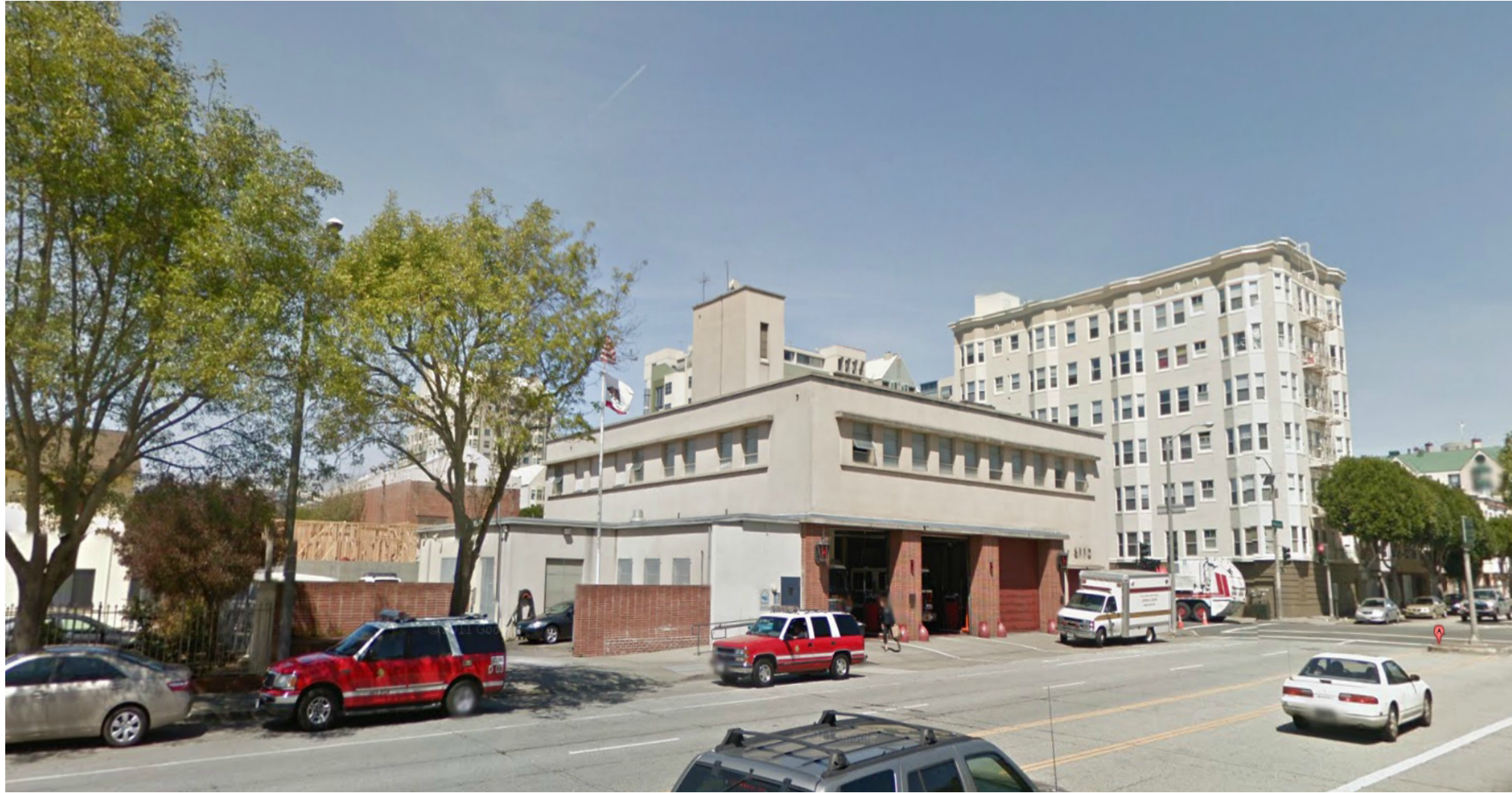
WEBSTER STREET - SOUTH & EAST FACADES
