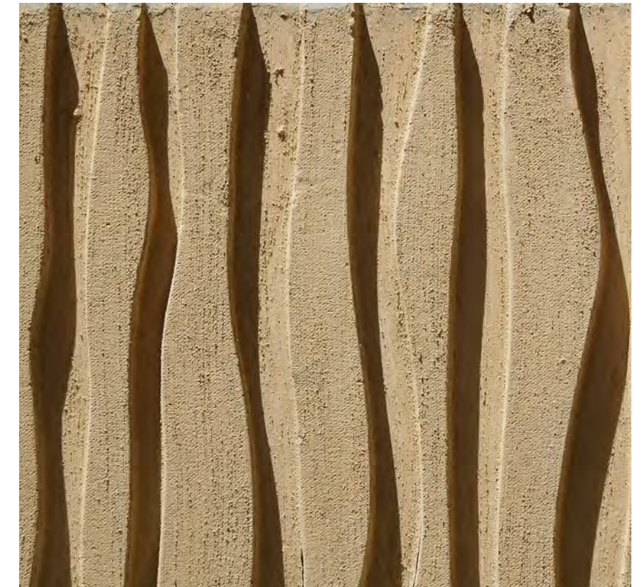
EXISTING CAST-IN-PLACE CONCRETE PATTERN
