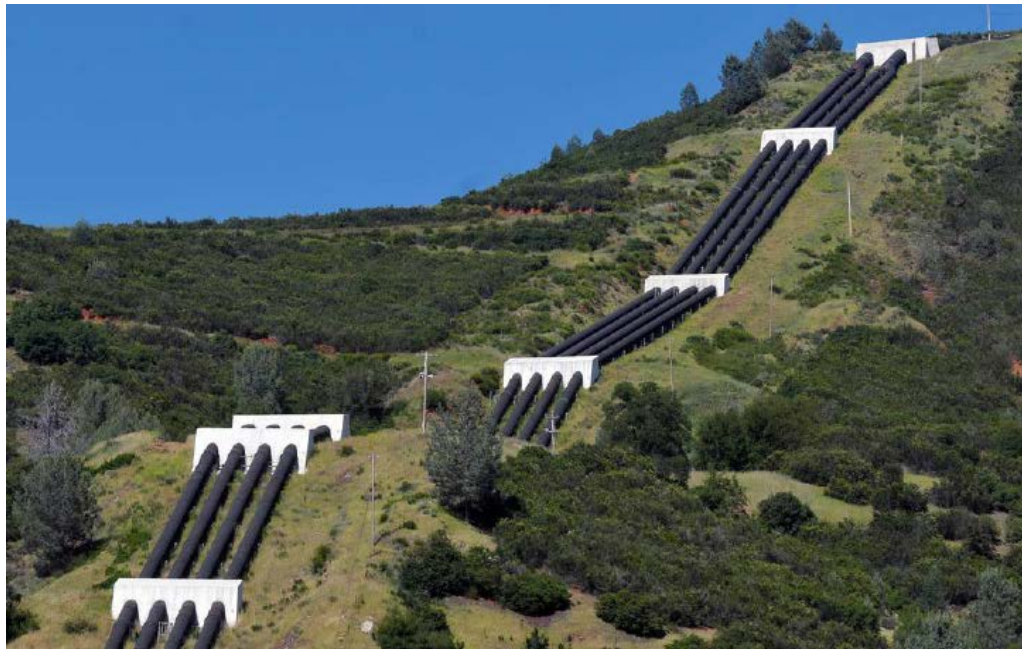
Water being piped in from Hetch Hetchy Reservoir to the New Power Plant
