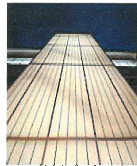
removeable kalwall roof system
