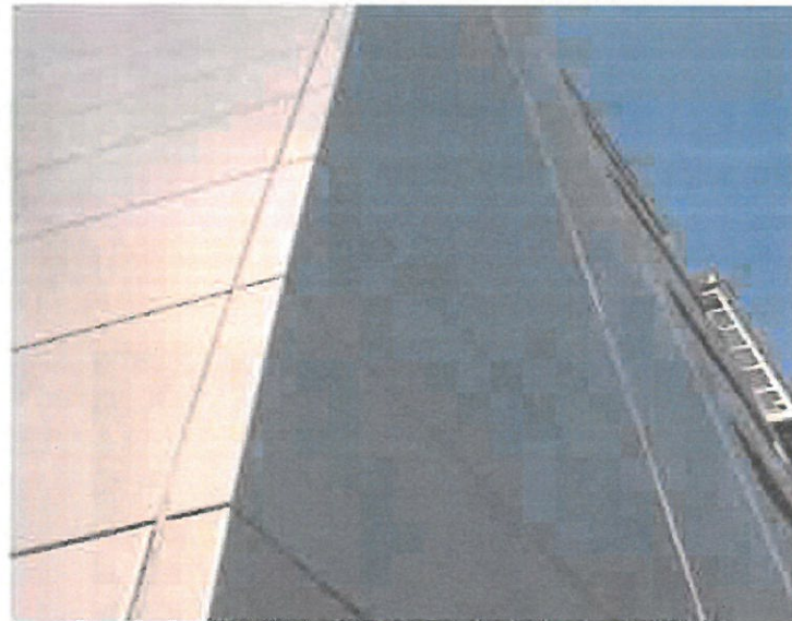
anodized aluminum wall panels and door cladding
