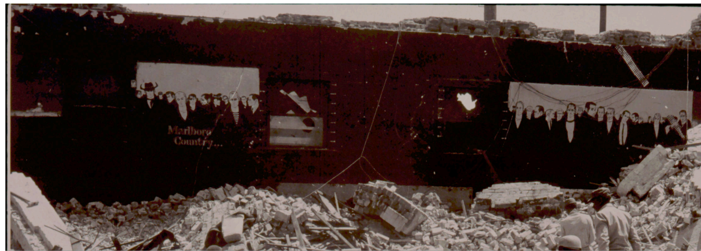
THE TOOL BOX & MURAL: MID DEMOLITION
