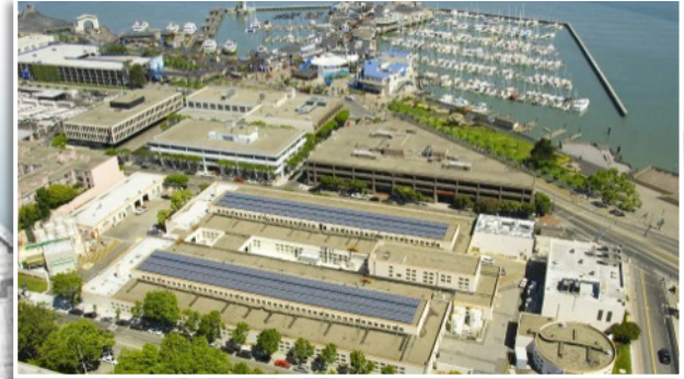
North Point Wet Weather Facility
