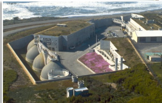
Oceanside Treatment Plant
