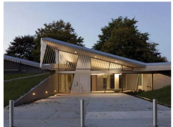
Water treatment facility, Portland
