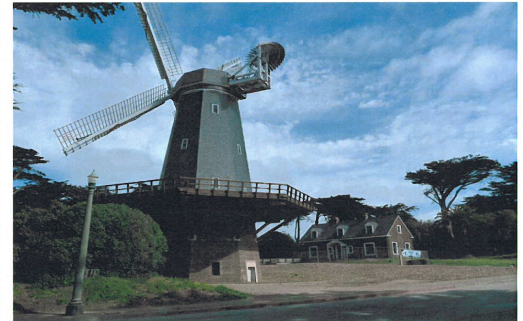
Murphy Windmill & Millwright's Cottage seen from MLK Jr. Drive
