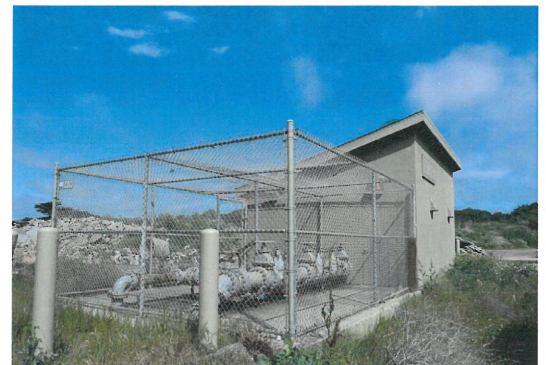
Southeast View Of Existing Well Station
