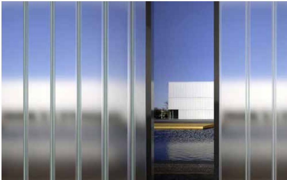
CHANNEL GLASS, NEW RESIDENCE AT THE SWISS EMBASSY, STEVEN HOLL, WASHINGTON D.C.
