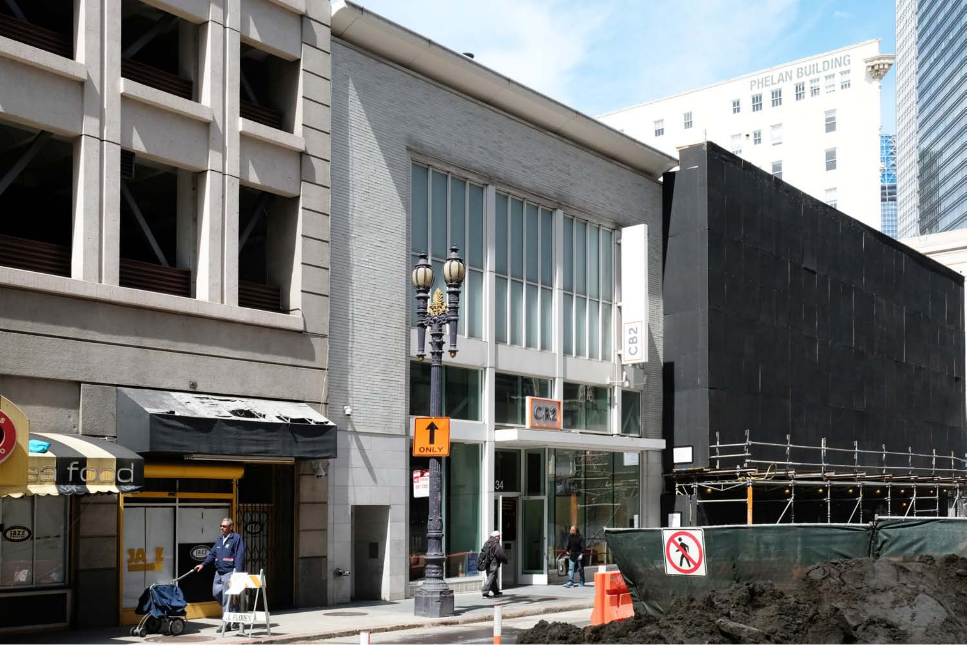
C. ELLIS STREET LOOKING NORTH EAST
