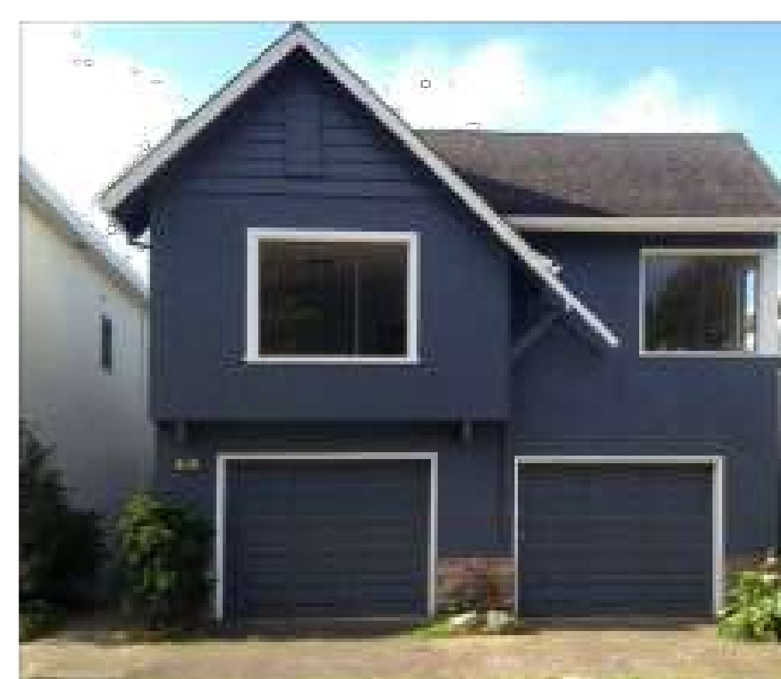
FRONT FAÇADE OF SUBJECT BUILDING
