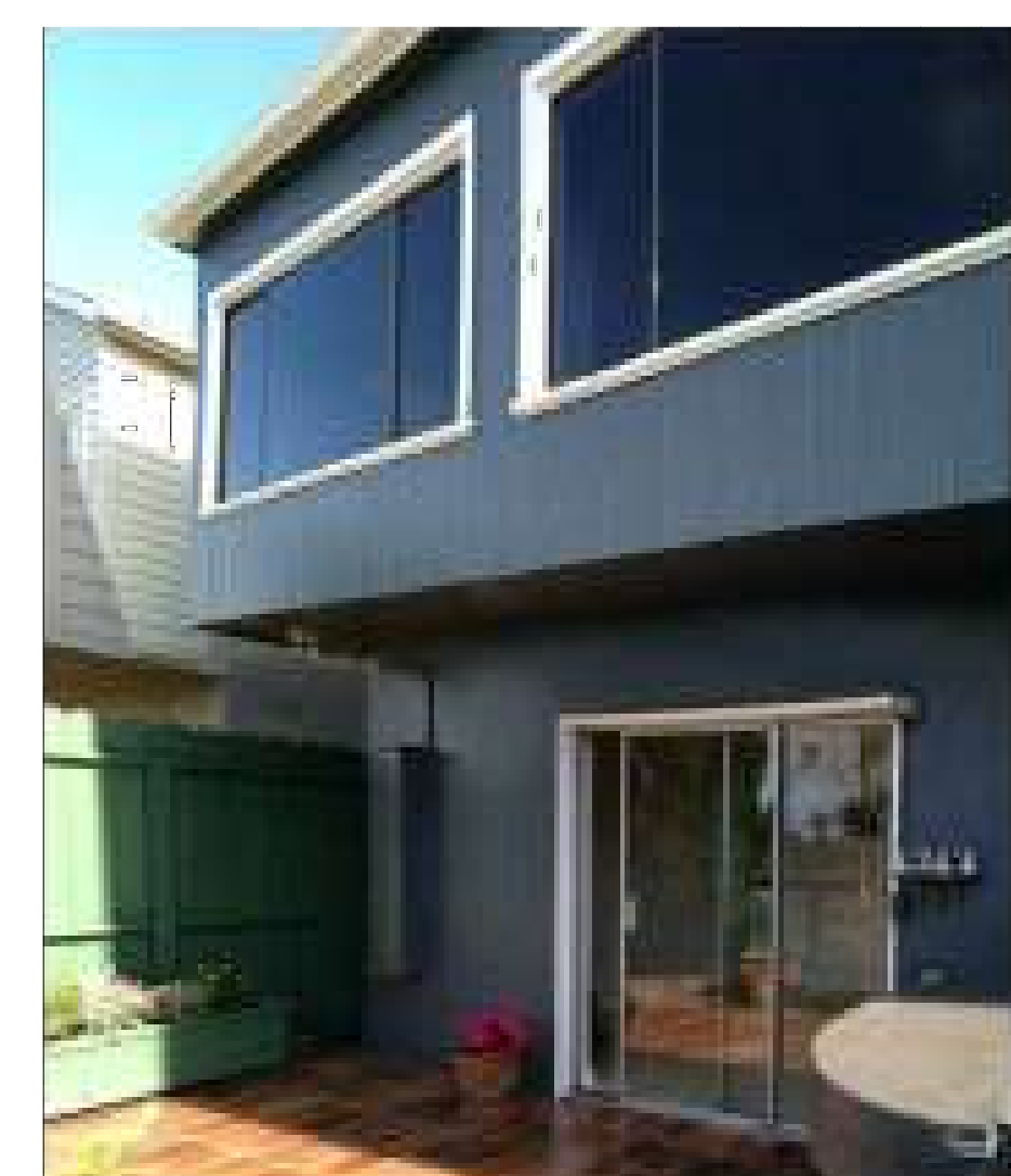
REAR FAÇADE OF SUBJECT BUILDING
