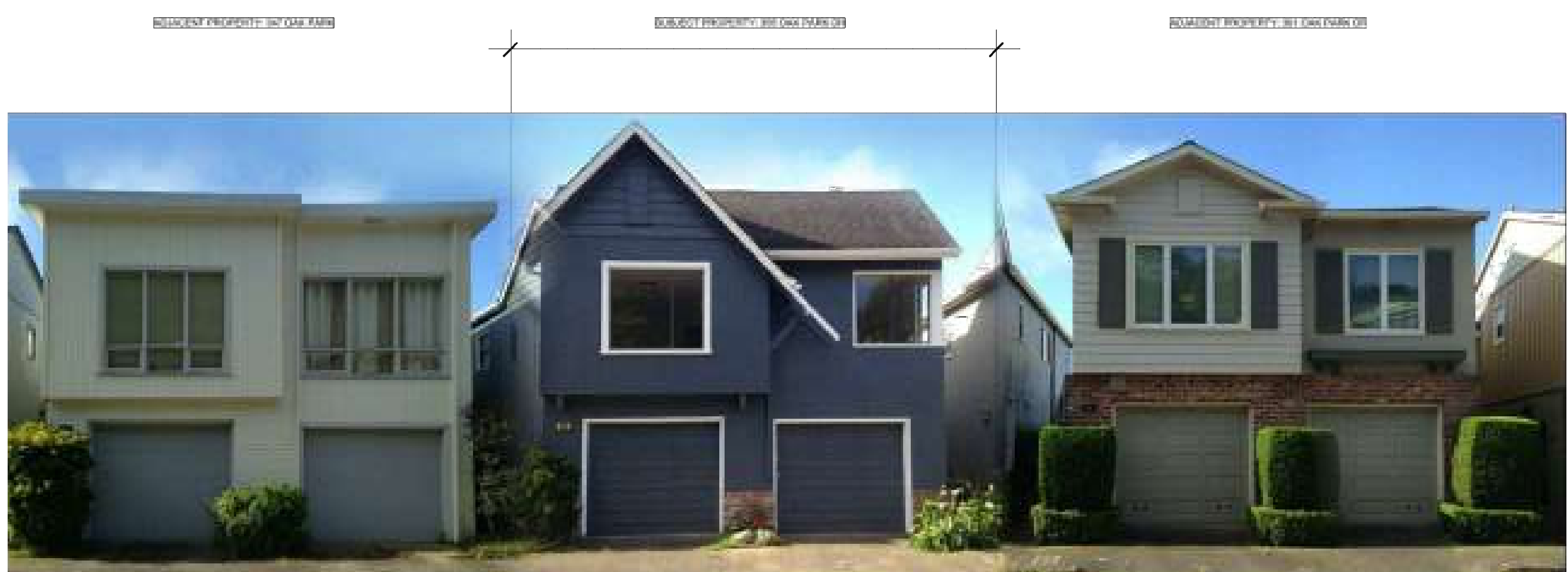
BUILDINGS ON SAME SIDE OF STREET
