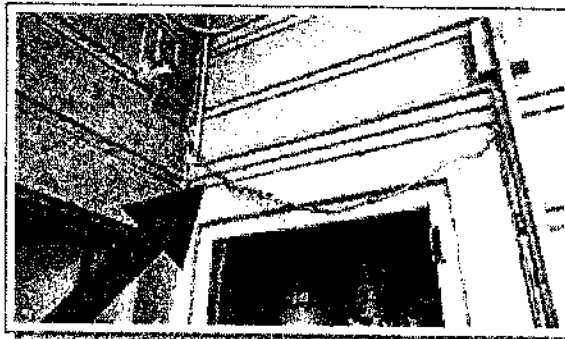
Exposed wiring - rear, pantry of unit 3431.
