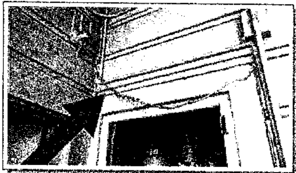
Exposed wiring - rear, pantry of unit 3431.
