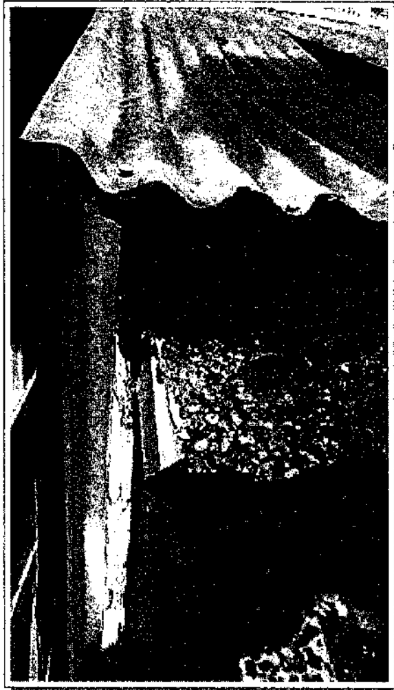
Decayed trim - right side wall at corrugated roof.
