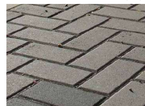
② PERMEABLE PAVING
