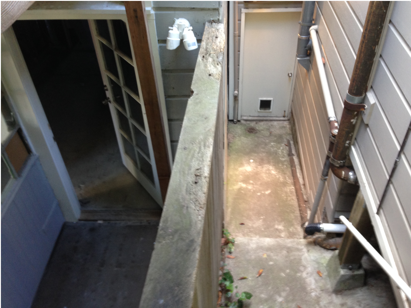
Photo of back of houses at 4121 and 4119 20th St.
