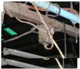
• In Building Two there is fluorescent lighting that has a broken conduit which exposes conductors. The cords to this lighting are hanging low which creates the risk of these cords being snagged.
