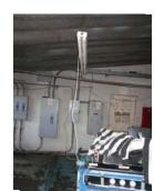
• Also in Building One, there is an overhead outlet box with open contacts that are exposed. Romex wiring was used inappropriately here. There is also an accumulation of combustible cloth fiber on an energized outlet.
