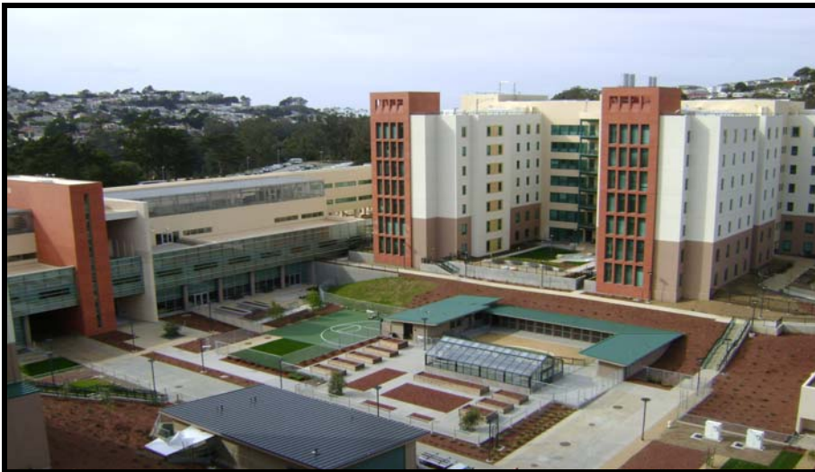
The Laguna Honda Hospital Replacement Program includes a healing garden (center) with ground level and raised beds, a greenhouse, and stalls for small animals.
