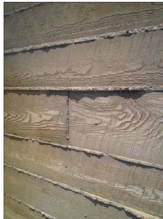
Board Form Concrete
