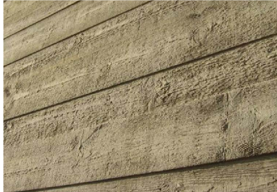
Board Form Concrete
