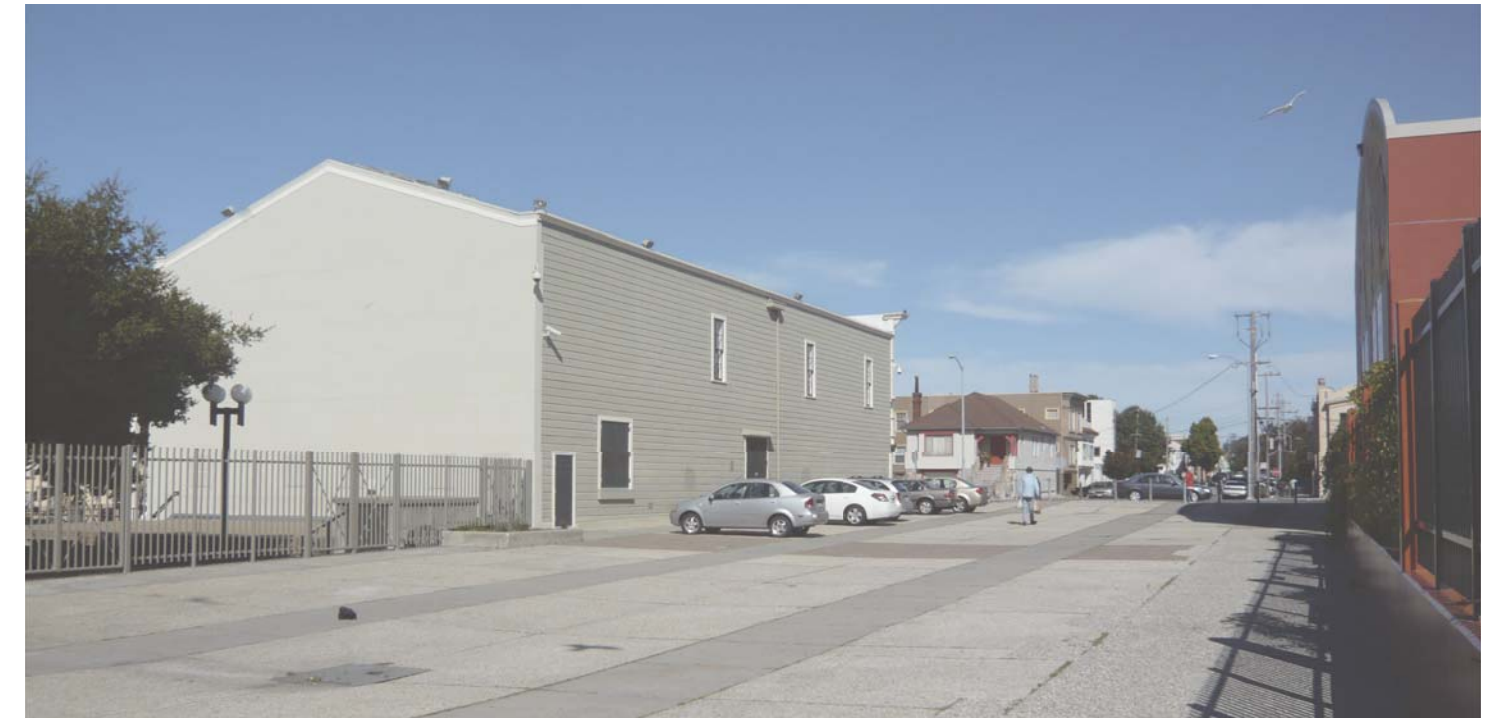
SOUTH SIDE OF OPERA HOUSE, PARKING LOT
