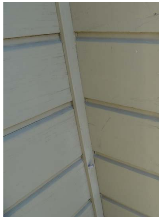
Existing 9" Exposed Face
