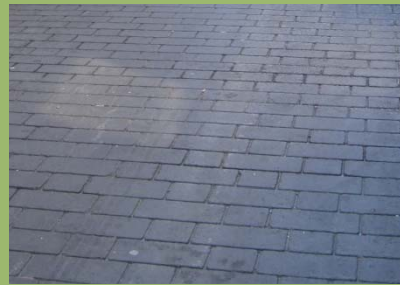
Asphalt Print Paving
