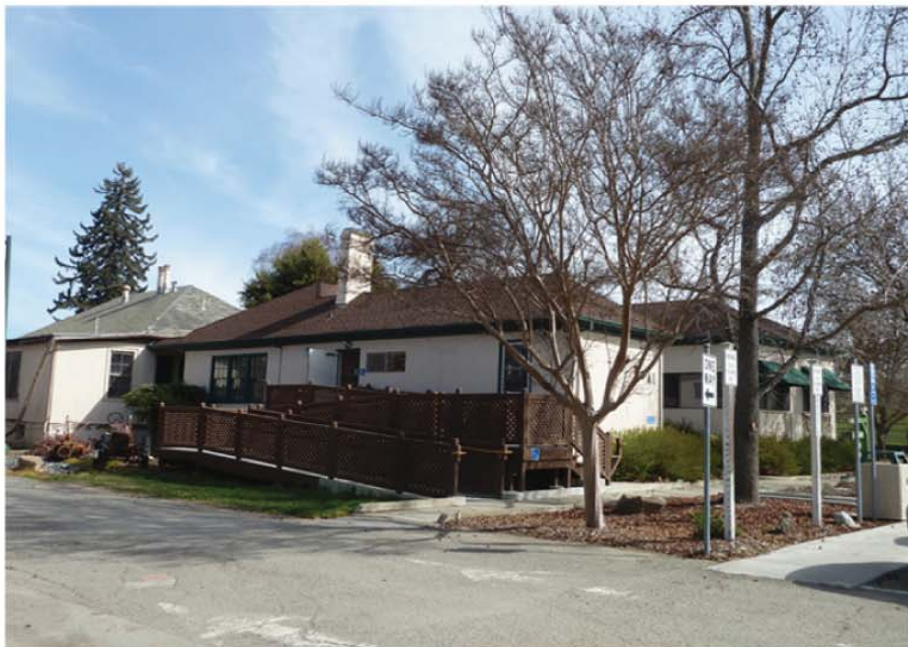
Existing Administration Building
