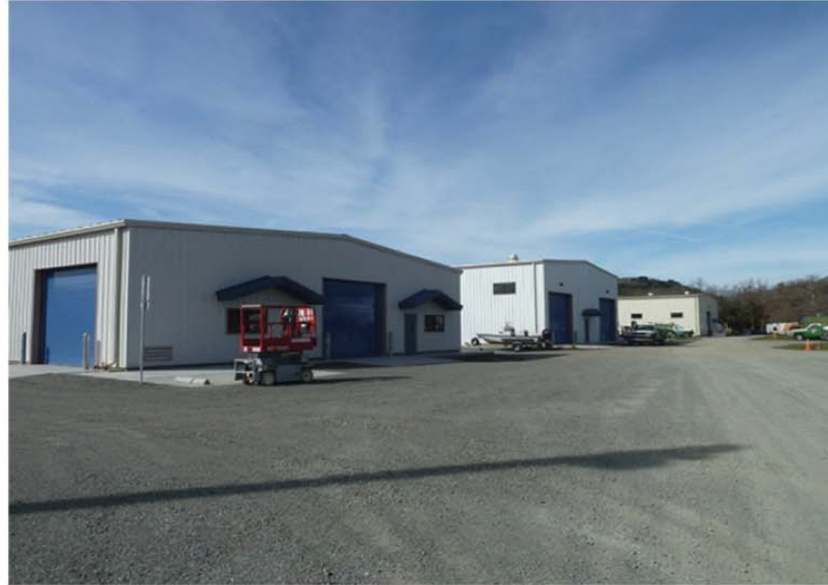
Existing Shop Buildings to Remain
