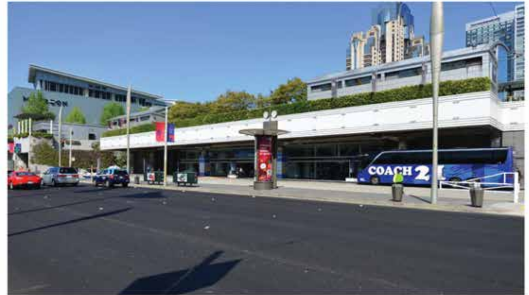
HOWARD STREET LOOKING AT NORTH LOBBY
