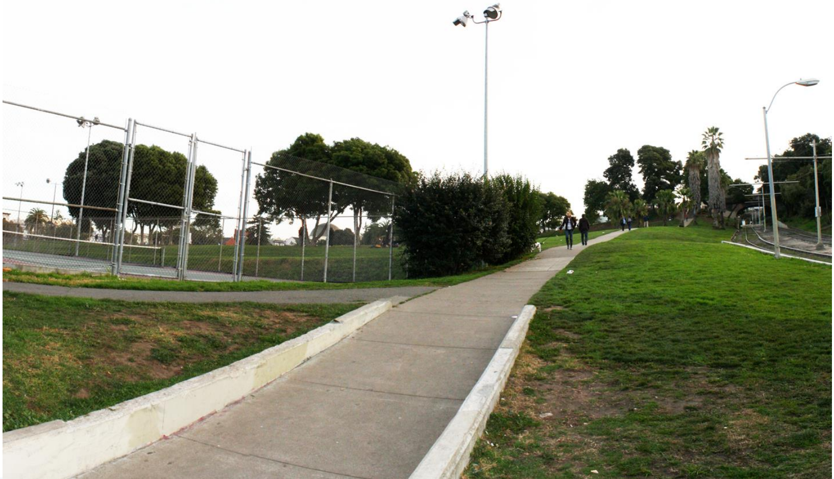
Existing Condition near 18 th / Church Streets
