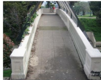
CONCRETE BRIDGE EXPRESSED CORNERS
