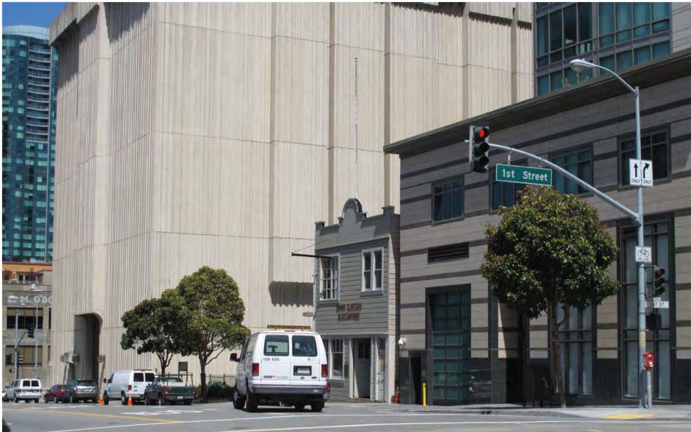
6 At First Street: view east down Folsom toward PG&E substation
