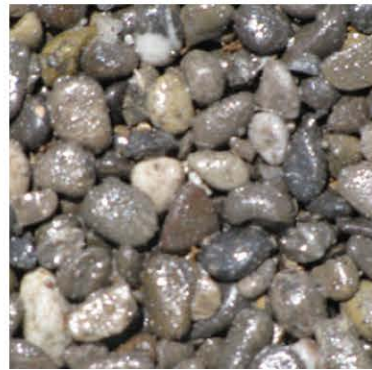
Resinset Gravel Chameleon Ways 5' x 8' area at street trees Addapave TP Dove Grey Pebbles
