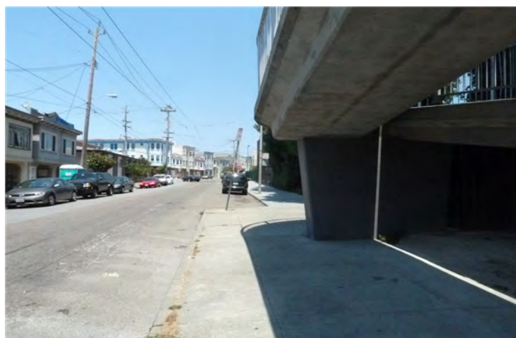
HAMPSHIRE ST. VIEW TOWARD NORTH
