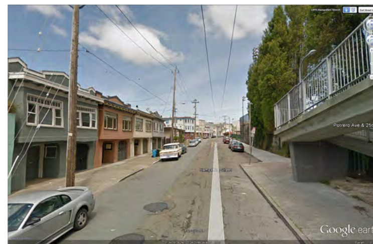
HAMPSHIRE ST. VIEW TOWARD NORTH
