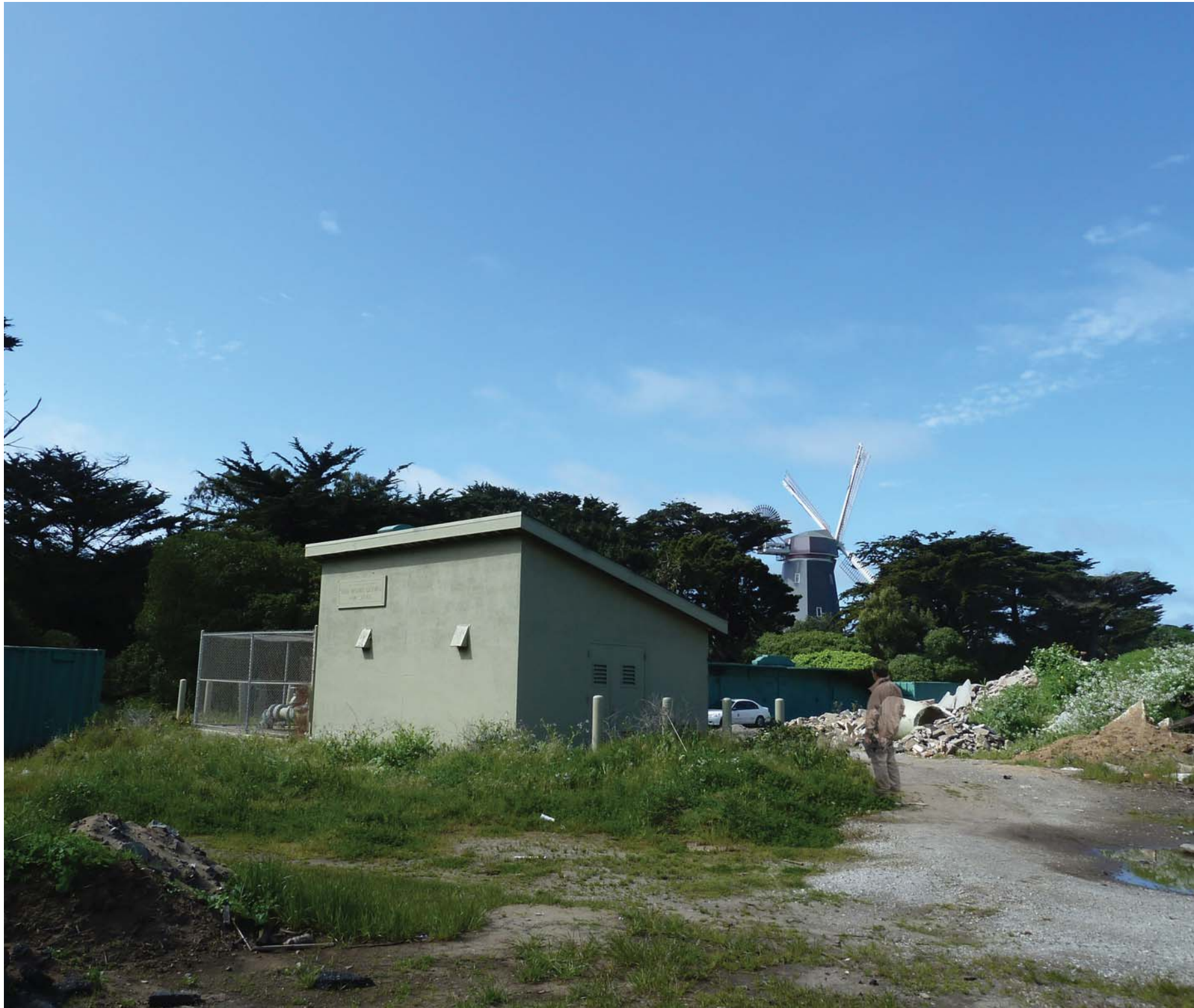
Northeast View of Existing Well Station
