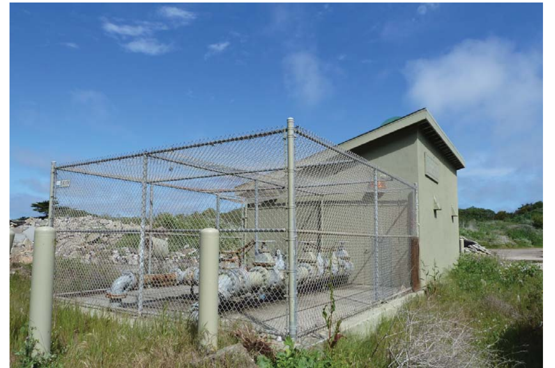
Southeast View Of Existing Well Station
