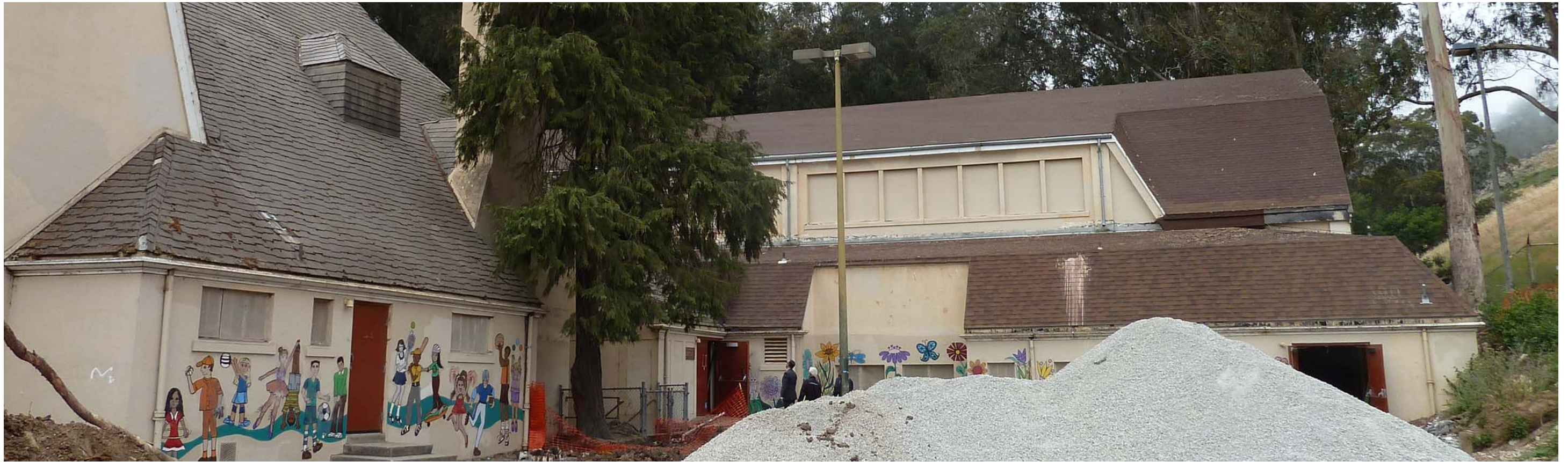
MAIN ENTRANCE - EXISTING PHOTO
