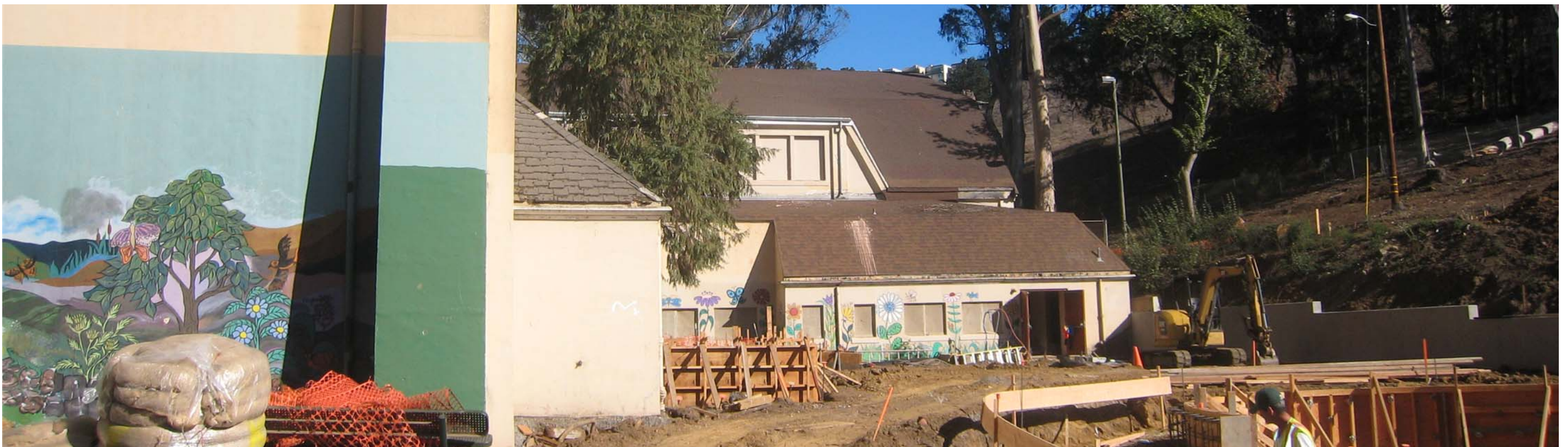
PATH TO ENTRY - EXISTING PHOTO
