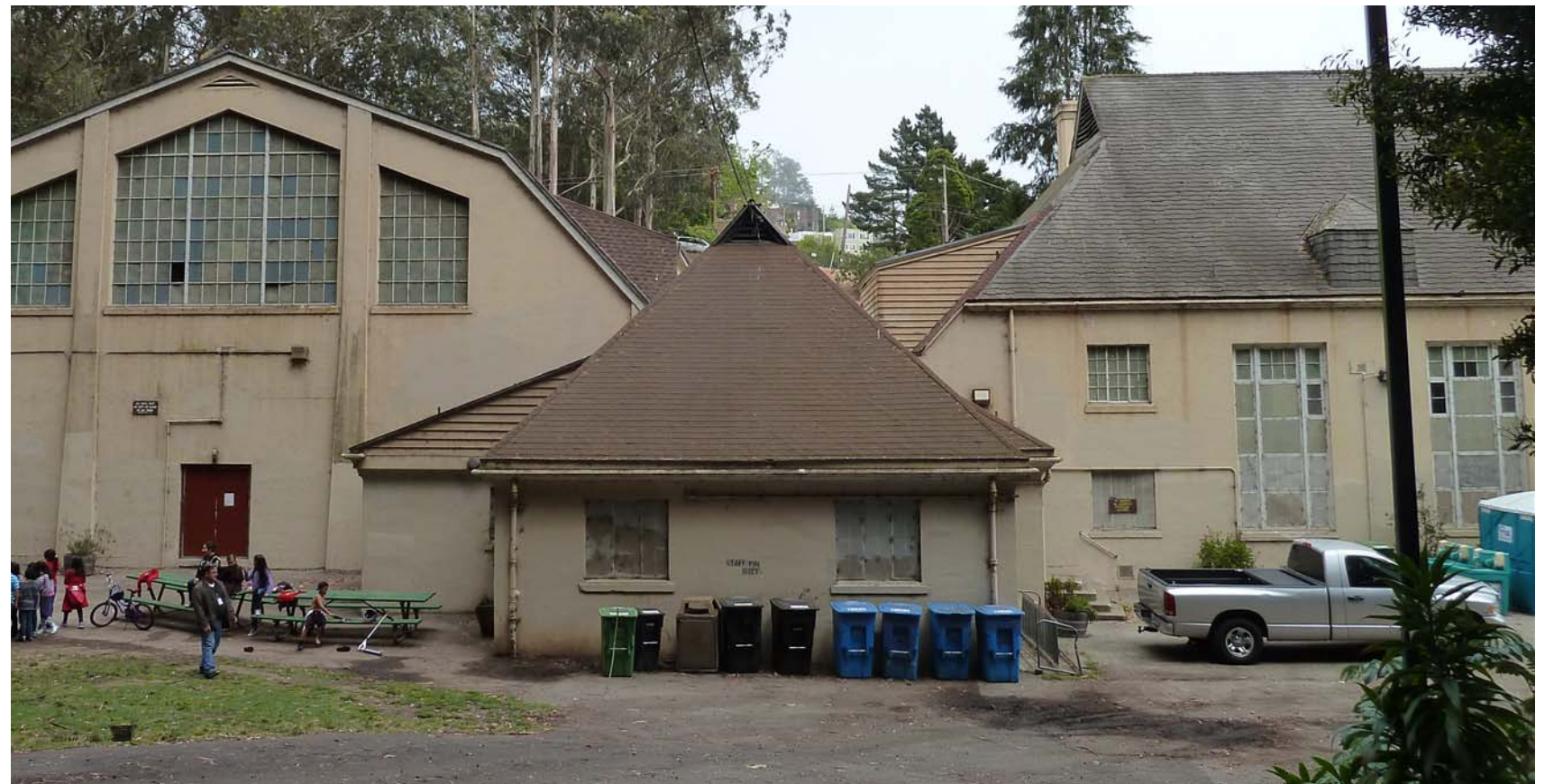
OFFICE WING - EXISTING PHOTO
