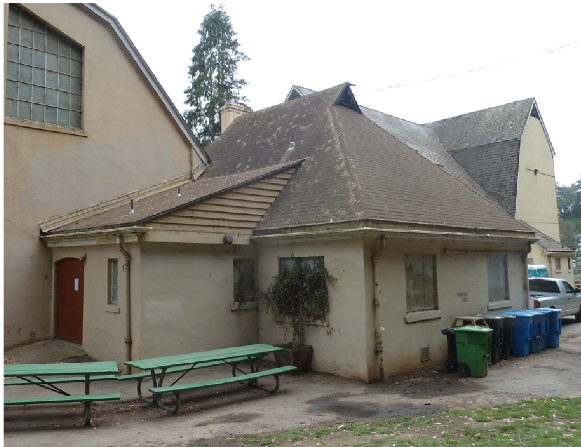
OFFICE WING - EXISTING PHOTO
