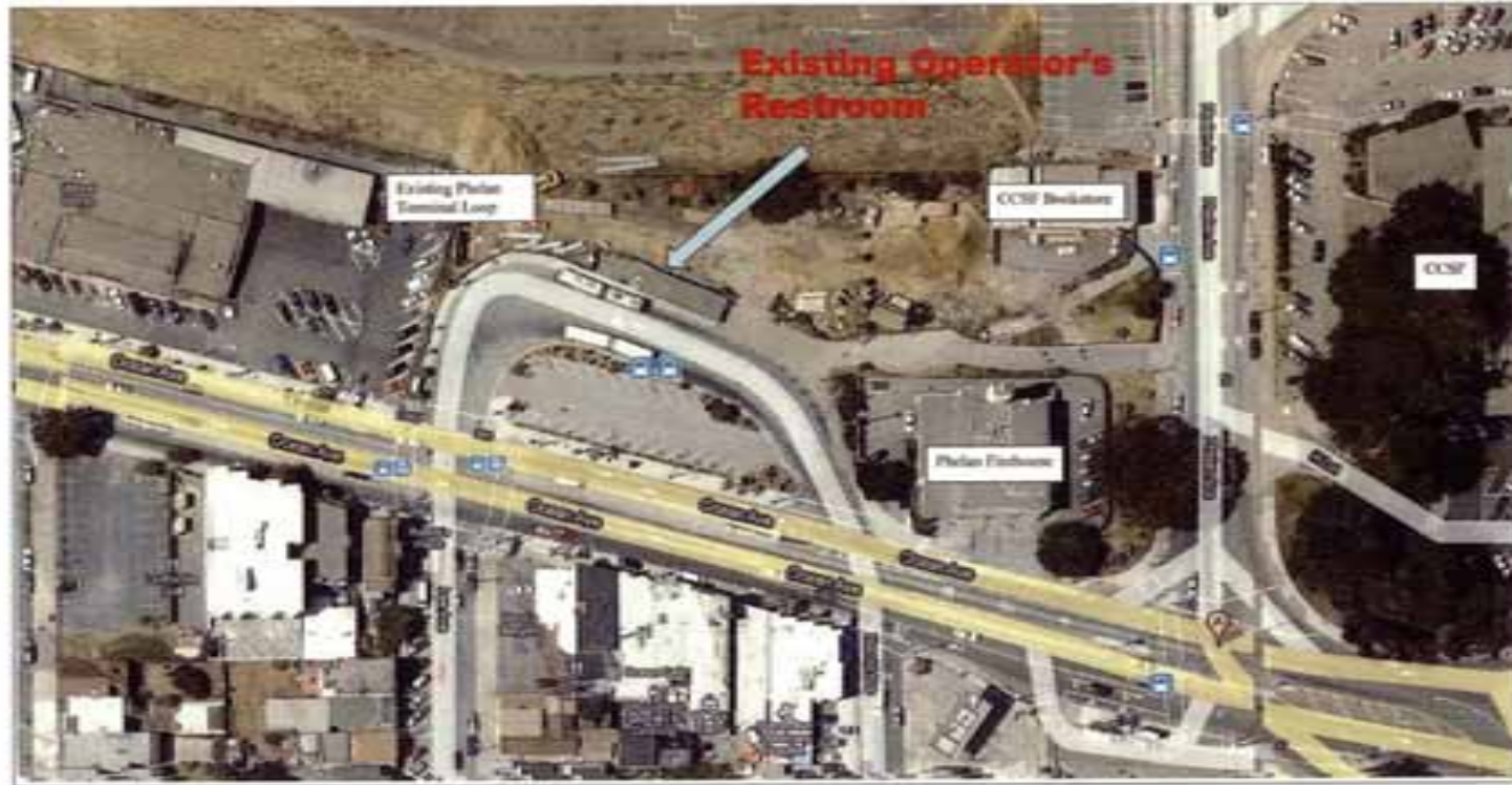
Aerial photo of existing Phelan Loop Area, 3/30/2010
