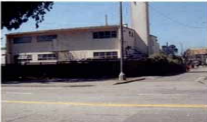
PHELAN AVENUE FIRE STATION
