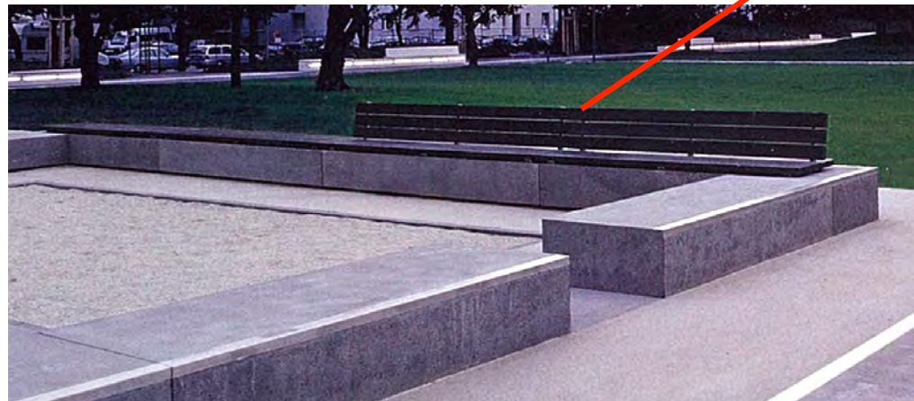
SEATING AREAS: Concrete, Steel with Wood seat and back, length of back and arm rests consistent with City requirements for public spaces.
