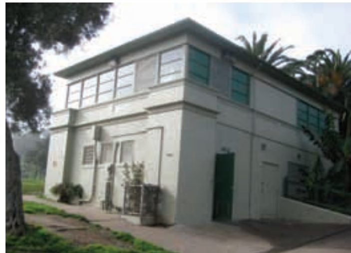
CLUBHOUSE ADDITION PRONOUNCED CORNERS + HIP ROOF
