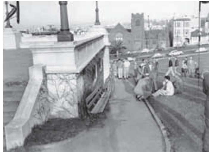
CONVENIENCE STATION - 1940'S CONCRETE FRIEZE
