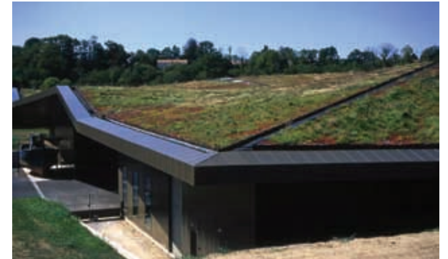
LOW SLOPE GREEN ROOF
