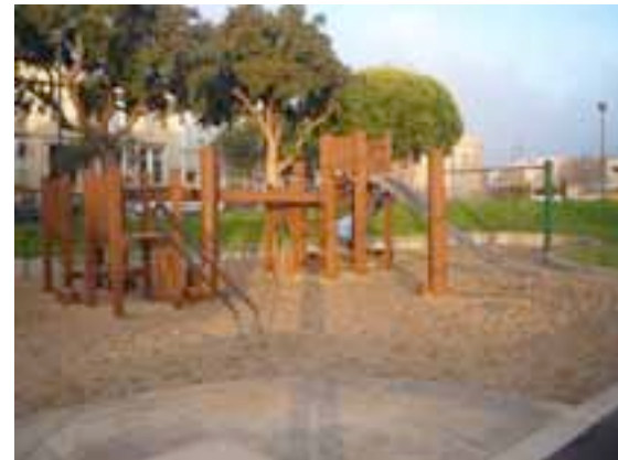
Older Play Structures (West View) Renovate Playground
