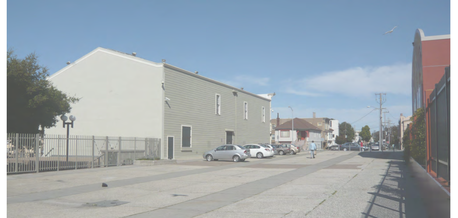
SOUTH SIDE OF OPERA HOUSE, PARKING LOT
