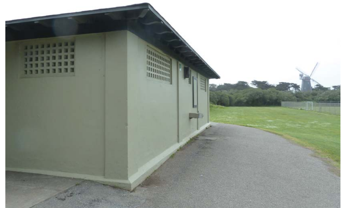
Northwest View of Existing Field House
