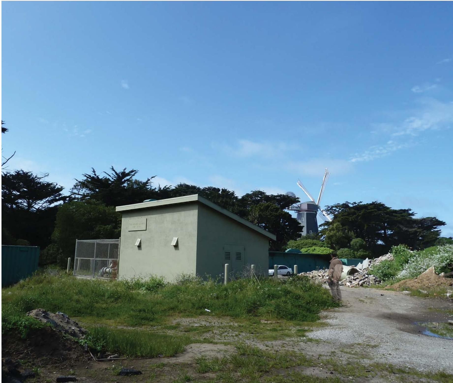
Northeast View of Existing Well Station
