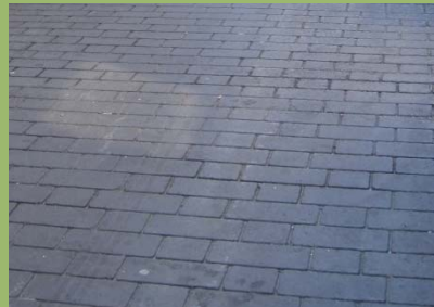
Asphalt Print Paving
