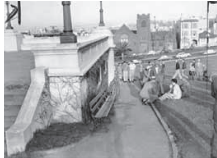
CONVENIENCE STATION - 1940'S CONCRETE FRIEZE
