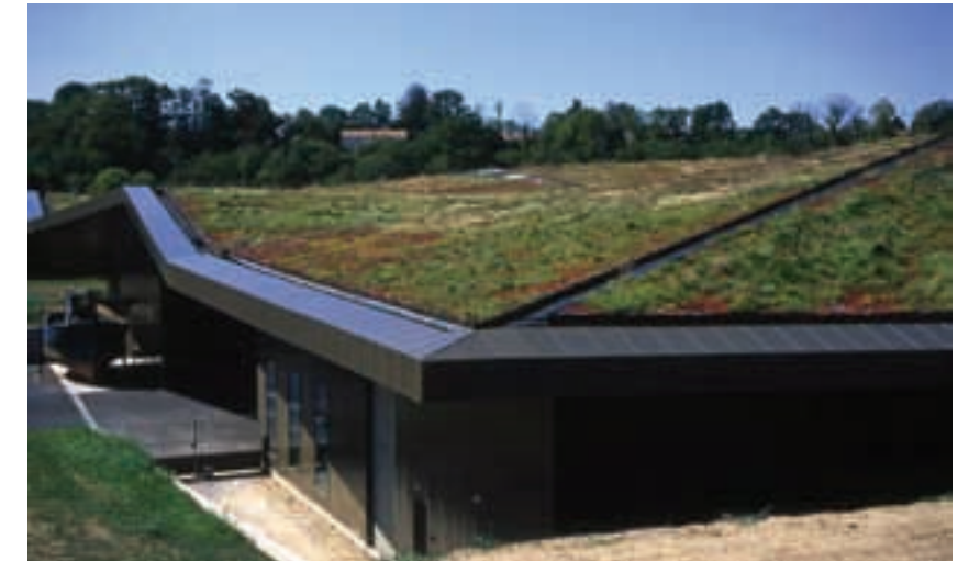
LOW SLOPE GREEN ROOF
