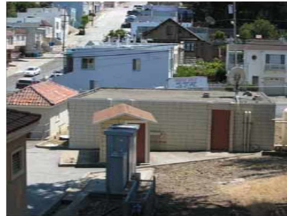
View of SFWD Pump Station
