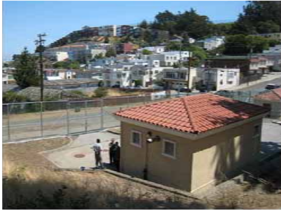
View of Rear Elevation-Generator Building
