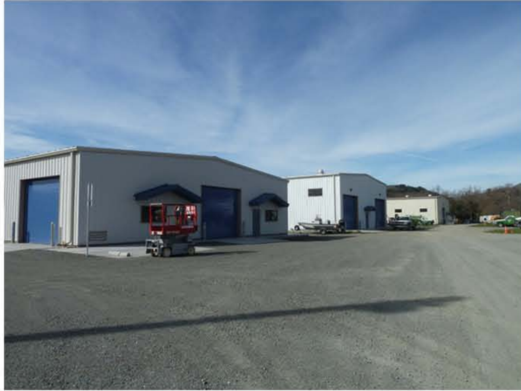
Existing Shop Buildings to Remain
