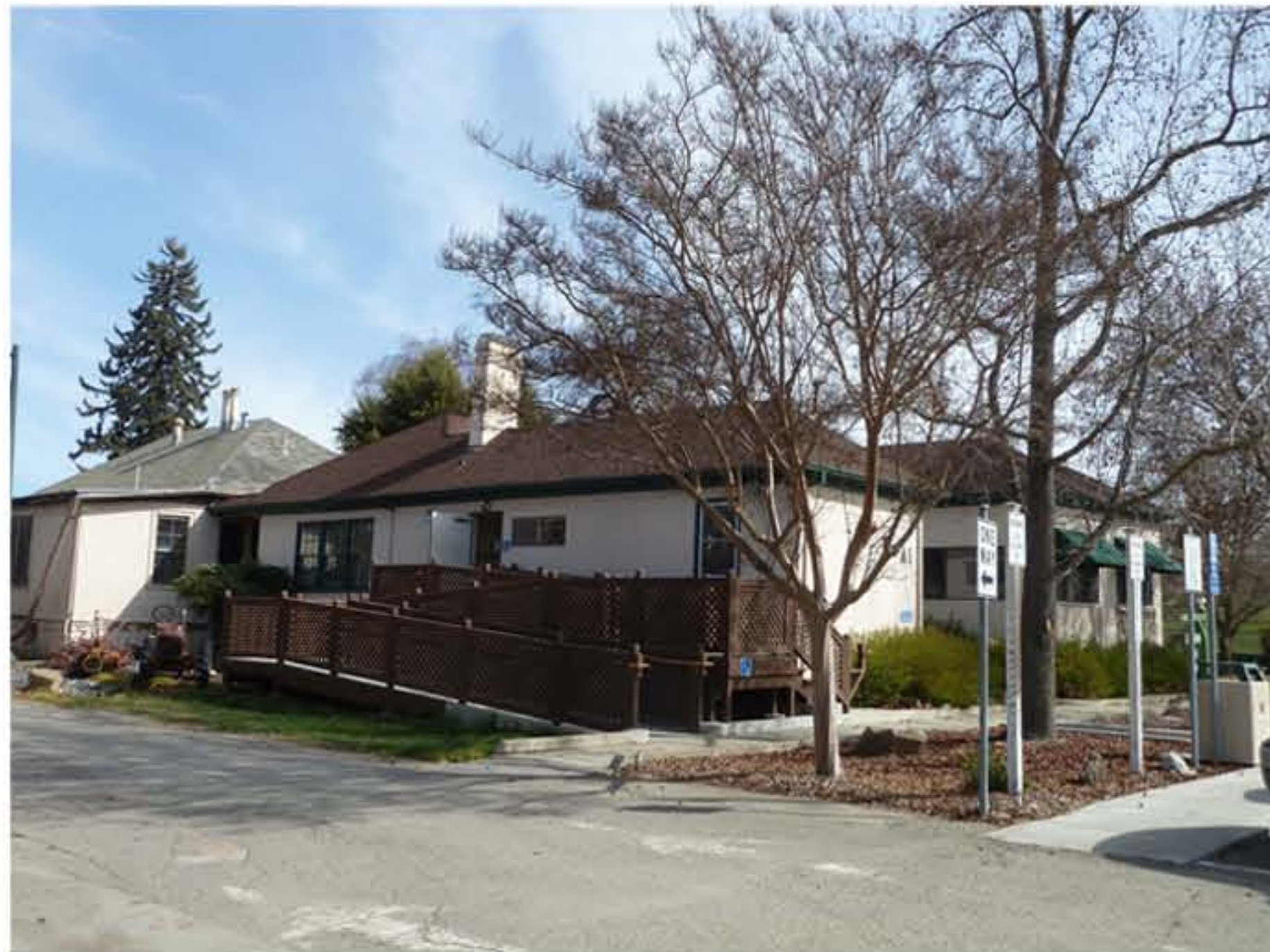
Existing Administration Building
