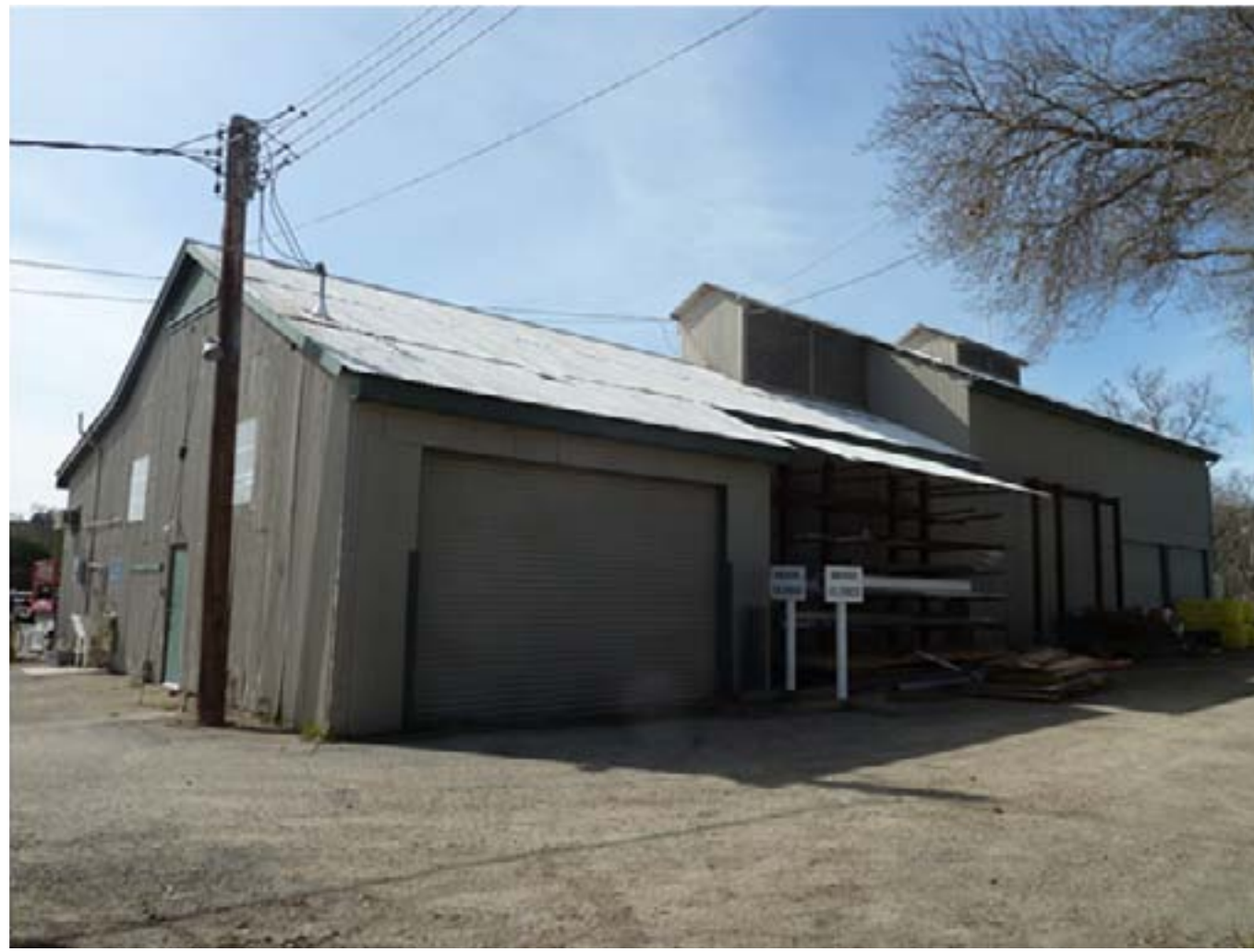
Existing Sunol Yard Buildings
