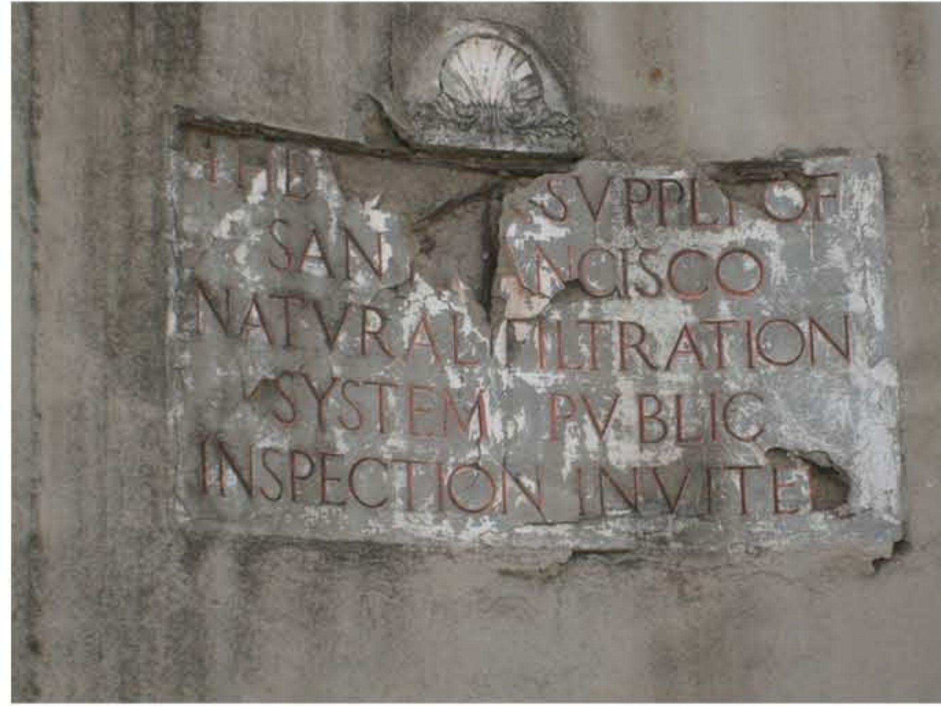
Main Gate Existing Condition Detail
