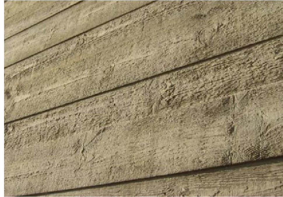
Board Form Concrete
