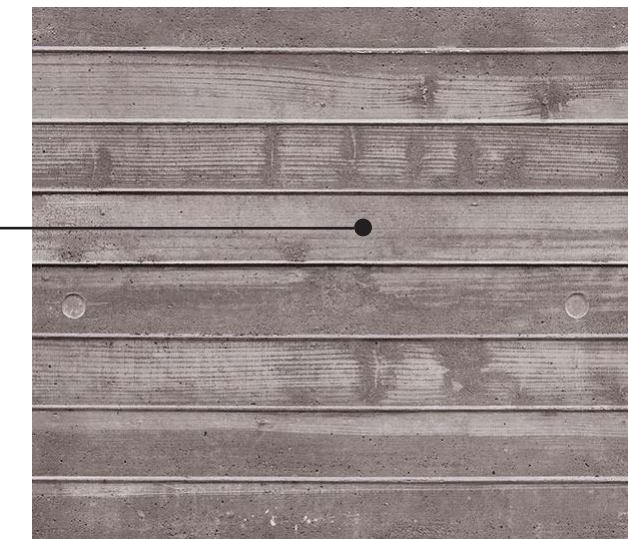
BOARD FORMED CONCRETE W/ SITE QUARRIED AGGREGATE
