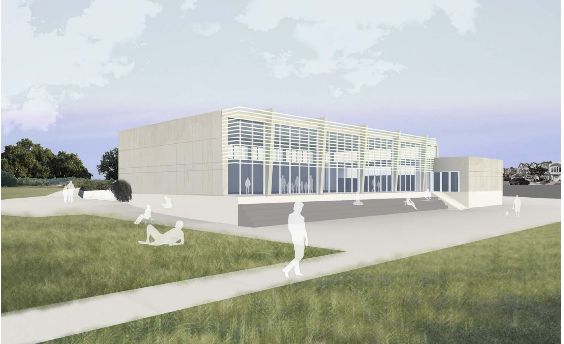
NEW WINDOW WALL AND SUN SHADE SYSTEM
