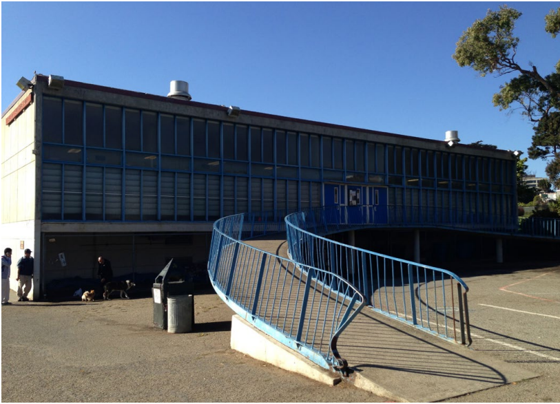
ENTRY EXISTING CONDITION
