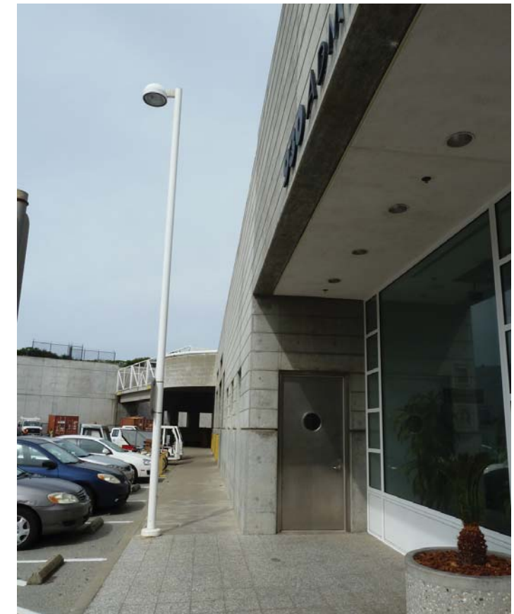
Existing Building Entrance
