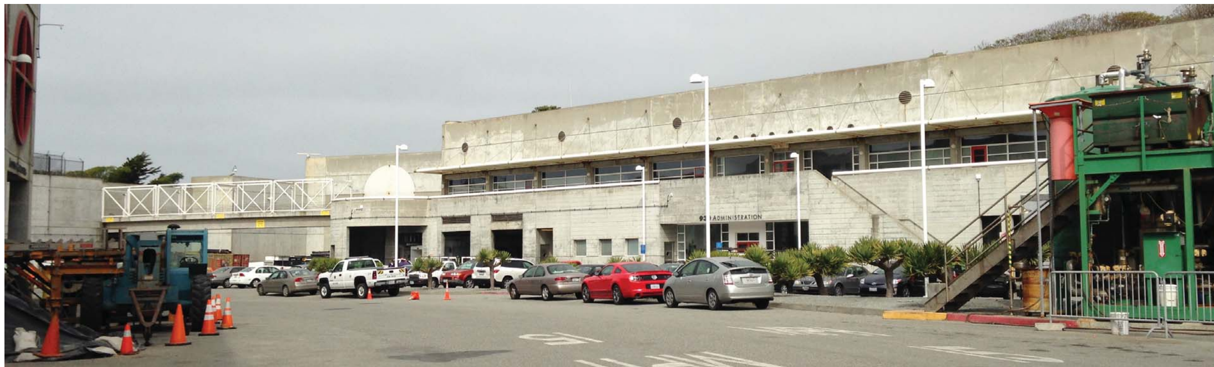
Existing Building Elevation
