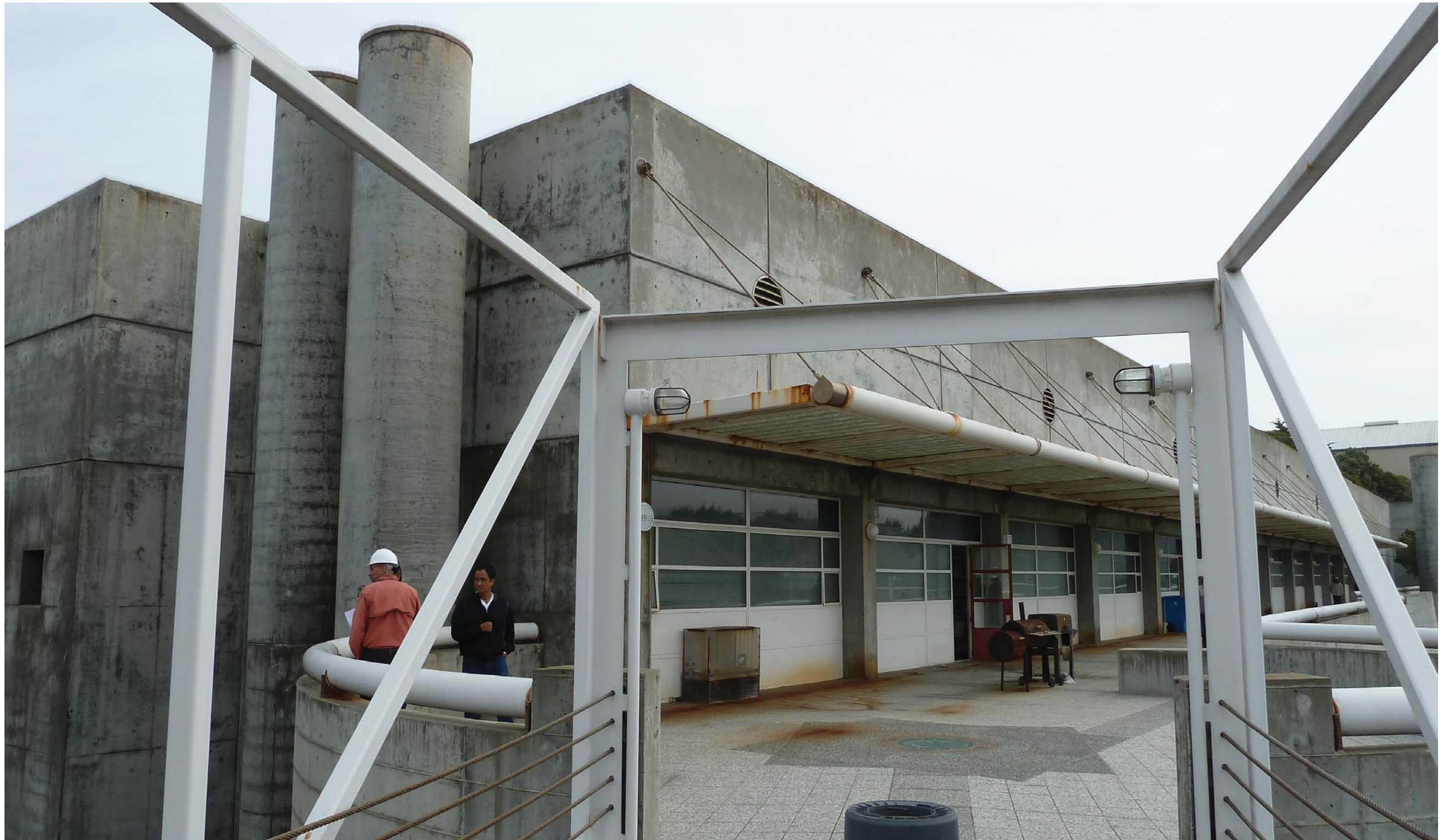
Existing Awning at Second Level Looking North-
