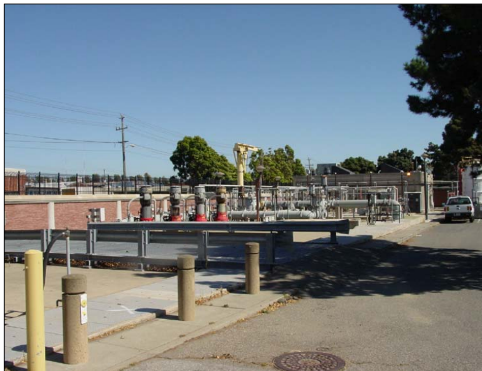
Photo Looking South towards Postchlorination Building
