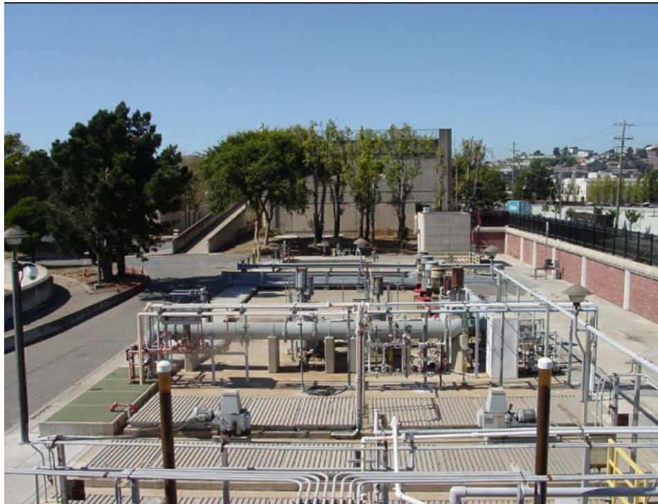
Photo Looking North at Equipment Yard
