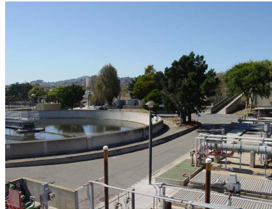
Photo Looking North-West towards Sedimentation Tanks
