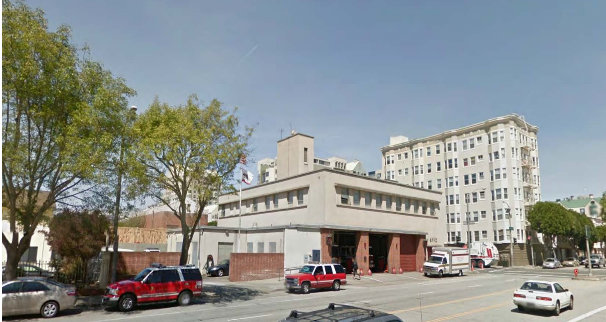
WEBSTER STREET - SOUTH & EAST FACADES
