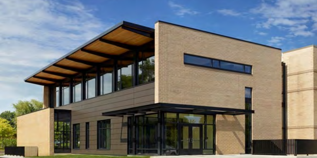
DUPAGE HOUSES OF WORSHIP CHAPEL & ADMINISTRATIVE WING - ILLINOIS
